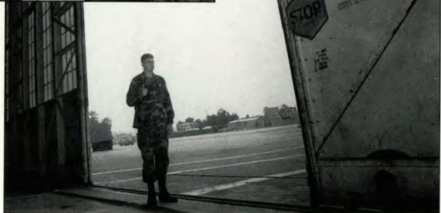
Hangar doors should never be opened to a width less than 10 feet. A spotter should always be used to ensure personnel and equipment are clear of doors.
